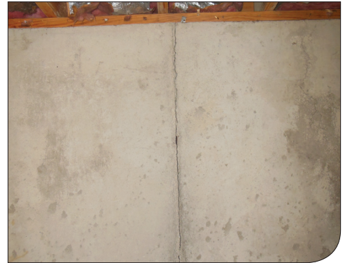
Vertical cracks
